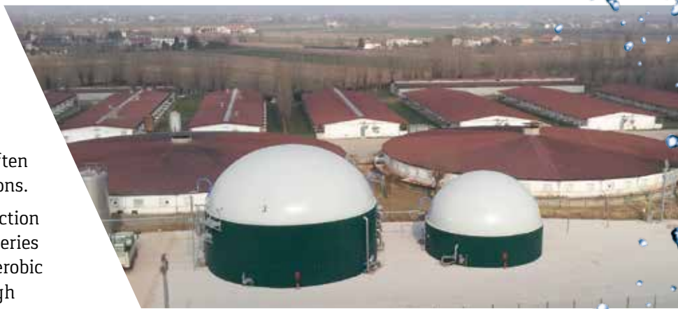
Anaerobic digestion plant of dairy by-products at Brazzale Dairy Farm in Campodoro, Padua, Italy.
